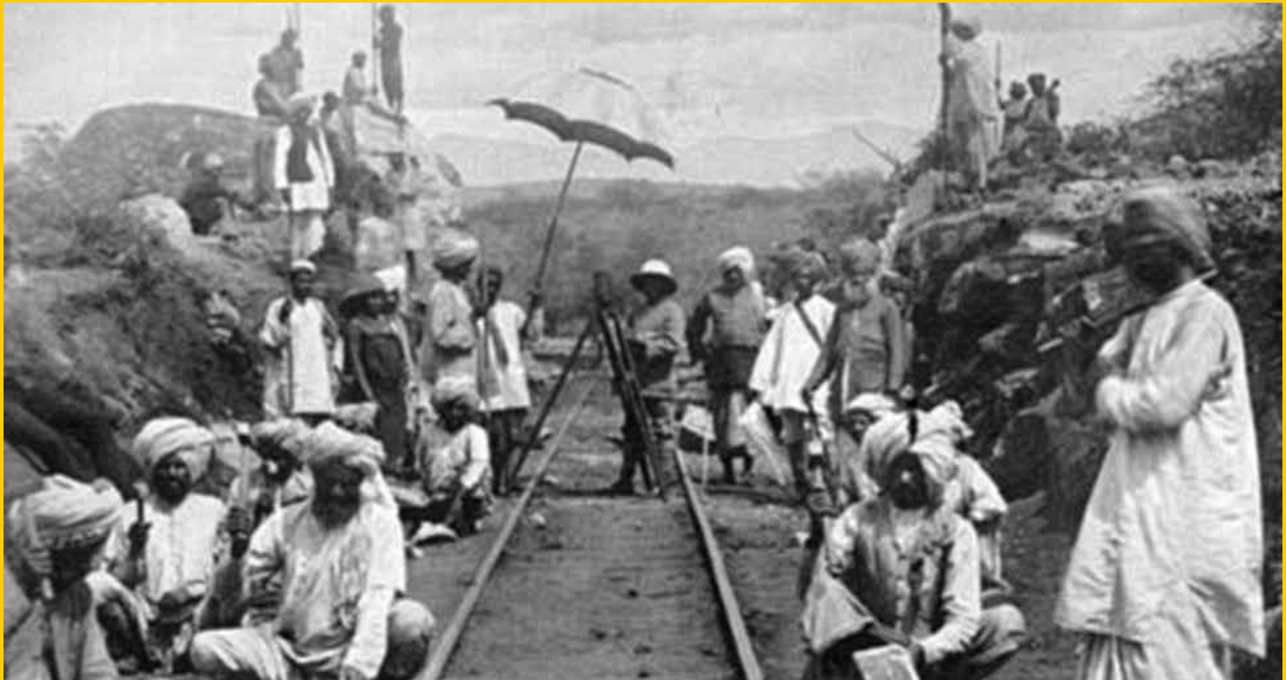
Indian Workers laying railway tracks in Kenya. More than 30,000 workers went from India to Kenya between 1896 to 1901.
